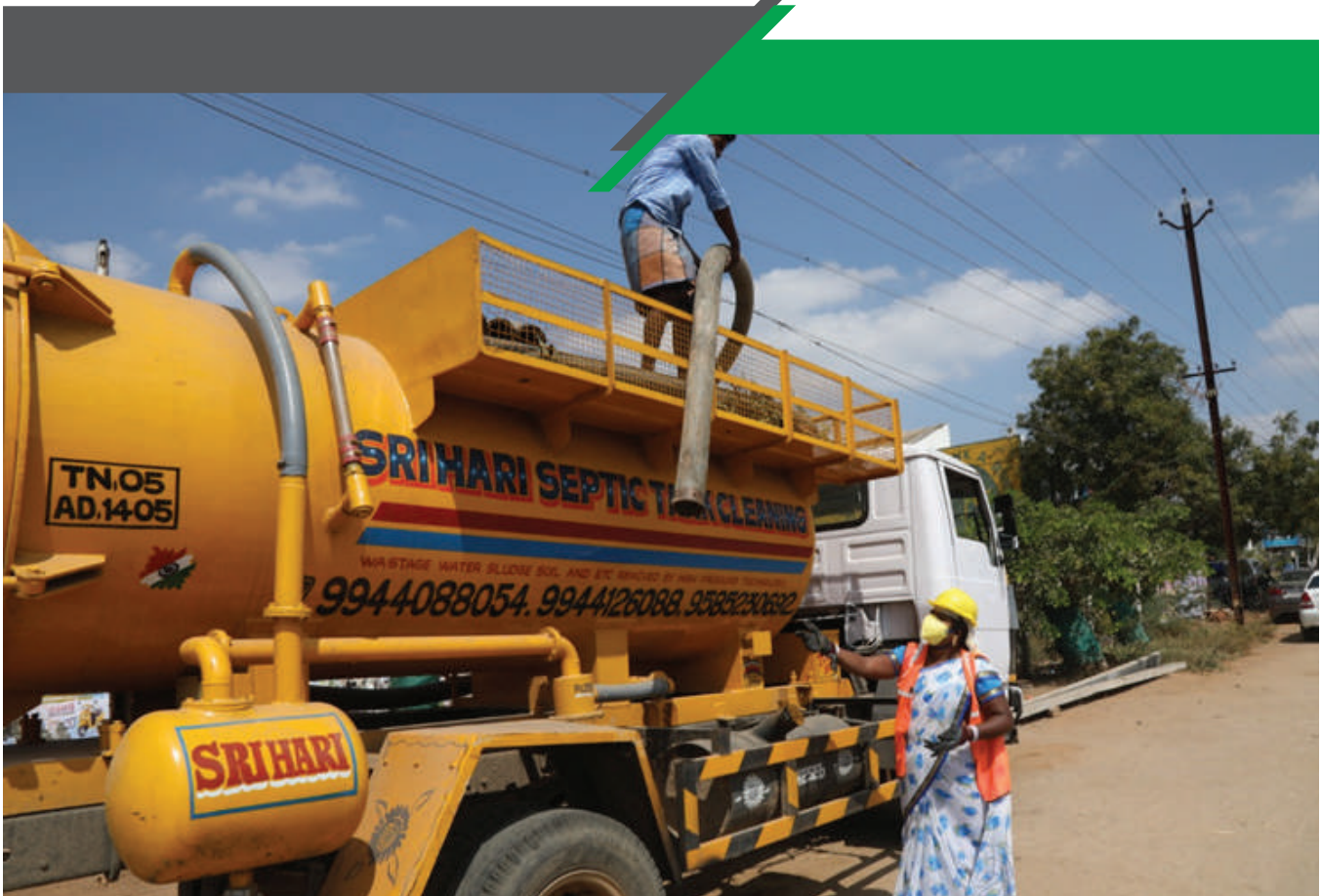
Trained sanitation workers involved in desludging septic tanks - Image Courtesy of NFSSM Alliance
