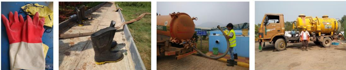
FIGURE 7: INAPPROPRIATE SELECTION OF PPE AS SEEN DURING SURVEYS
