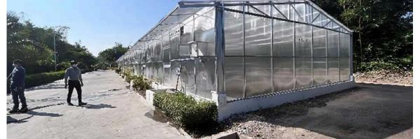
Solar drier effectively reduced the pathogens in sludge, making the sludge safe to use as manure/fertiliser
