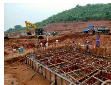
Figure 9: A plant under construction in Odisha
